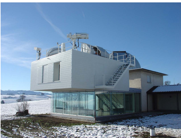
Figure 4. The new observatory for H 2 O located at Zimmerwald close to Bern.
